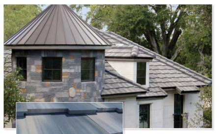
Installing a staggered exposure can seem daunting to an installer that has not done one before. The truth is that it is really quite simple. It just requires planning. The first thing to think about is waste. Remember, that approximately half of the tiles on the roof will have a shorter exposure than the other half. It will be essential to calculate that difference prior to ordering the tile.
