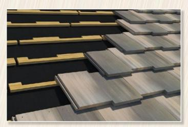
especially on steeper roof pitches where a majority of the face of each tile will be visible. If desired, exposed channel can be removed using a saw and/or tile nippers (as seen in lower inset illustration).
