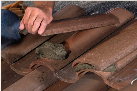
Placing The Mortar
