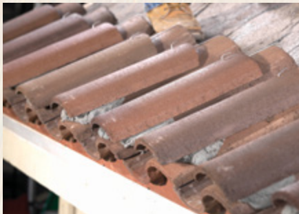
Boosting The Eave
