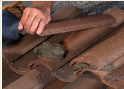
Placing The Mortar
