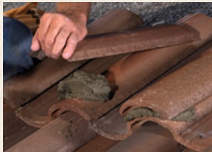
Placing The Mortar
