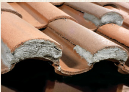
Close-Up of Boosted Eave
