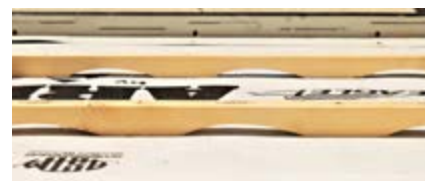
OPTIONAL BATTENS WITH SCALLOP OR OTHER DRAINAGE DESIGNS
